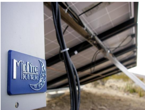
Left: Combiner installed on A pole mount array.
